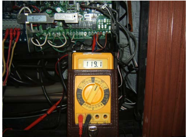
b) 115 VAC at the APM terminals on the control box.
